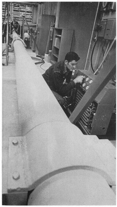
INSIDE BLDG. 882 the long air gun barrel is slung as a multiple pendulum to absorb a slight amount of the energy when fired. At right is C. W. Ray (7322-2) who is checking operation of the air compressor prior to a test shot. Compressed air under 5000 lbs. pressure per sq. in. powers the air gun At the breech end of the gun stand H. D. Sivinski (7311) and H. R. Bowers (7322).
